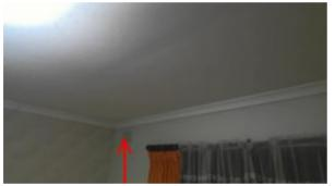
Cornice Damaged cornice Minor Defect Cornice has cracked and requires filling and repainting. (Painter)
