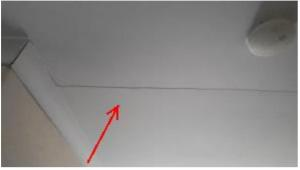
CeilingsDamage ceilingMinor DefectCeiling is damaged and requires repairing and repainting. (Painter)
