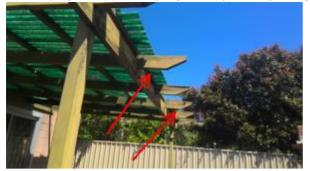
Roof coverDamaged roof coverMinor DefectType: AThe alsynite roof sheeting is damaged and requires replacing. (Roof plumber)
