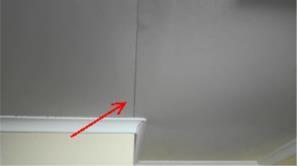
Ceilings Sagging Minor Defect Type: A Sagging has occurred to the ceiling, which requires re-fixing, filling and repainting. (Ceiling fixer & Painter)
