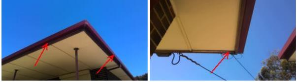
Gutters Gutters blocked with leaves and Minor Defect Type: A debris
